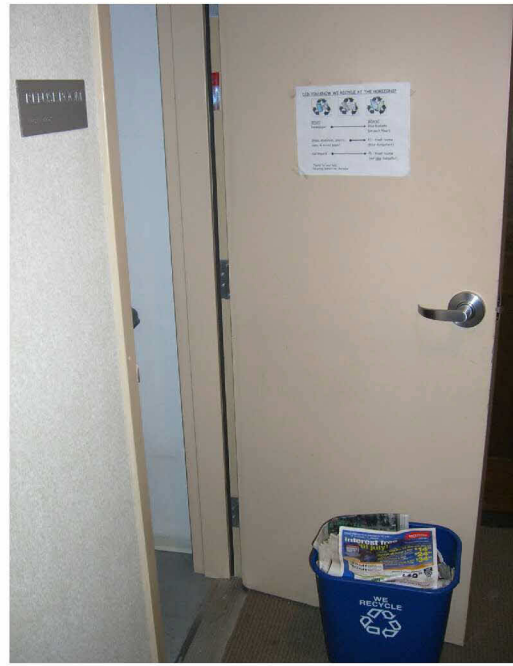
Newspapers and trash are transported by janitorial staff to the Garbage & Recycle Rooms beneath each tower.
